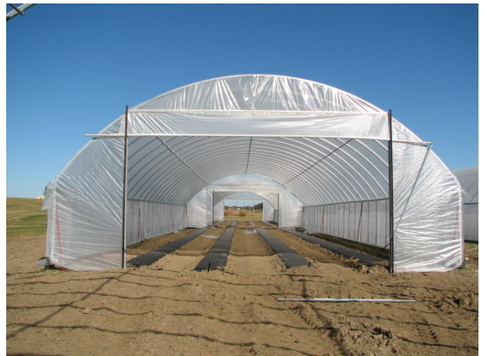
One of five new 30' x 96' high tunnels ready for planting at Mississippi State University's South Research Farm.
